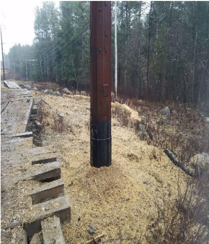
Fig 7: Exposed soils mulched with straw at Str. 53. Viewing southeast. (03-13-20).
