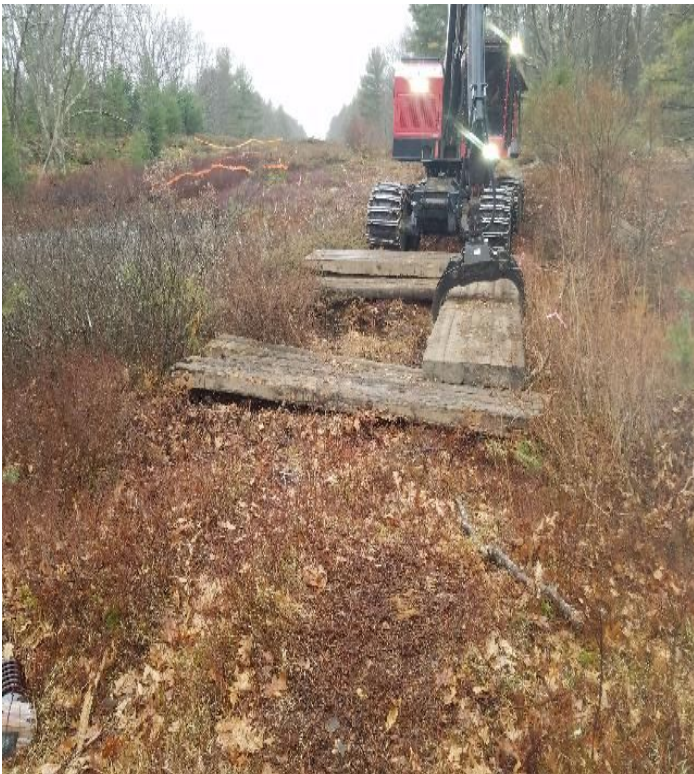
Fig 23: Beginning to bridge over wetland DW40 between Strs 80 and 81. Viewing west. (03-17-20).
