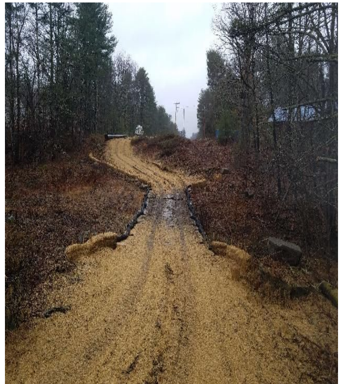
Fig 12: Access road through wetland DW48 Viewing west. (03-13-20).
