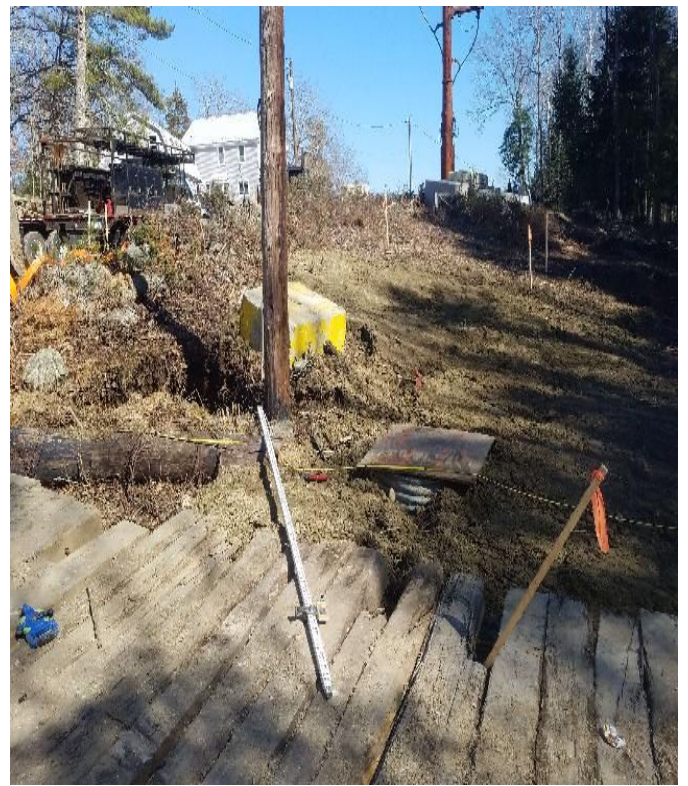
Fig 28: Excavating foundation for Str. 98. Viewing east. (03-18-20).
