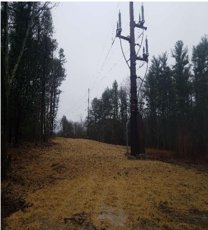
Fig 15: Exposed soils mulched with straw at Str. 100. Viewing east. (03-13-20).
