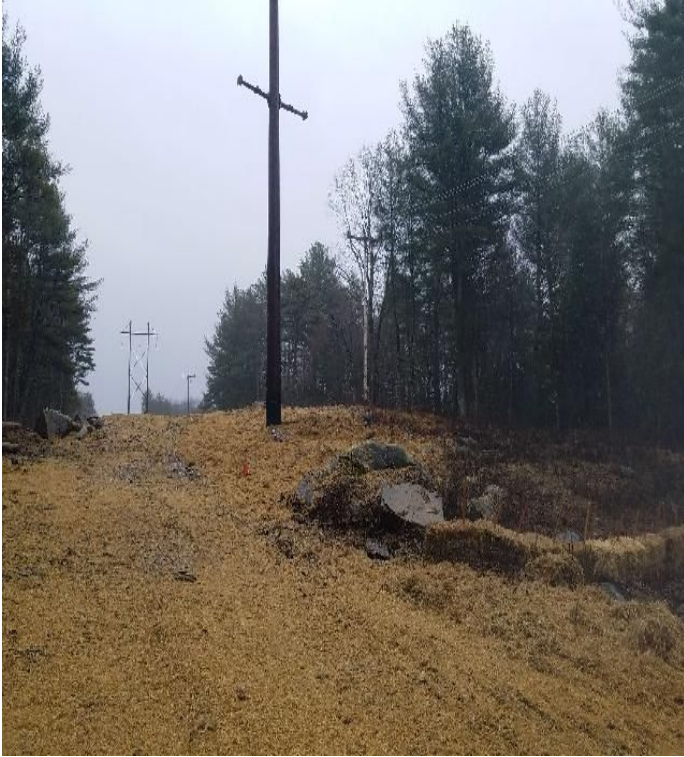
Fig 9: Exposed soils mulched with straw at Str. 55. Viewing east. (03-13-20).
