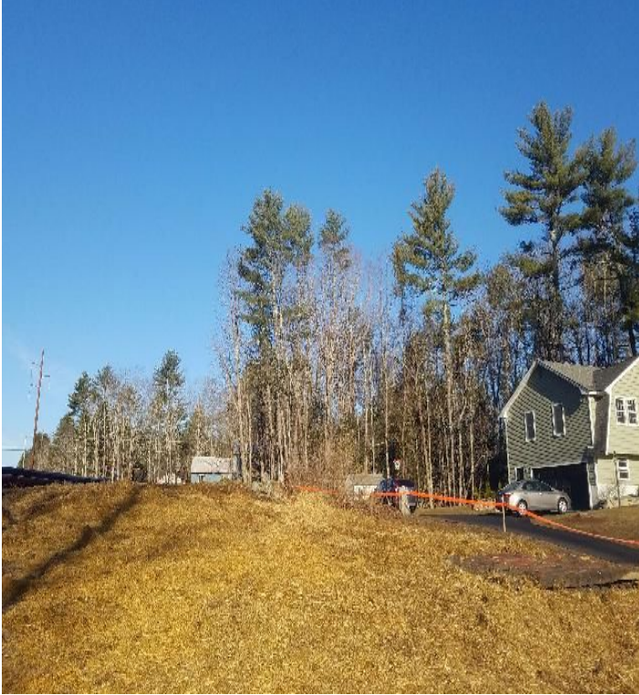
Fig 25: Exposed soils mulched with straw at Str. 67. Viewing west. (03-18-20).
