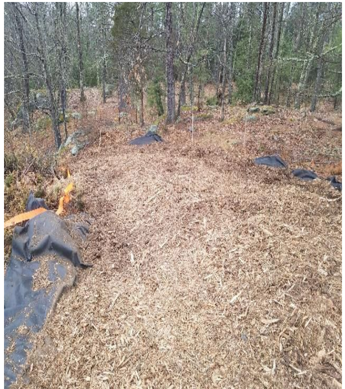
Fig 24: Stump grindings applied to off-right-of-way access between Strs 79 and 80. Viewing northwest. (03-17-20).
