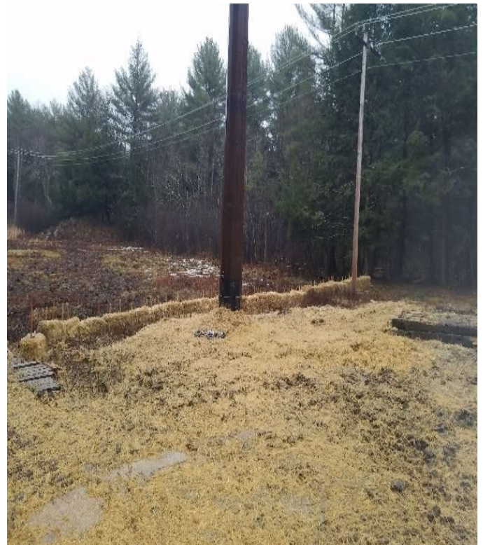
Fig 8: Exposed soils mulched with straw at Str. 54. Viewing east. (03-13-20).
