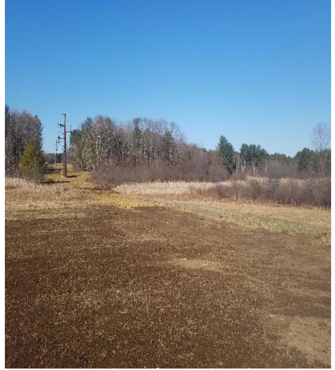
Fig 26: Removing timber mats at Frink farm. Viewing west. (03-18-20).
