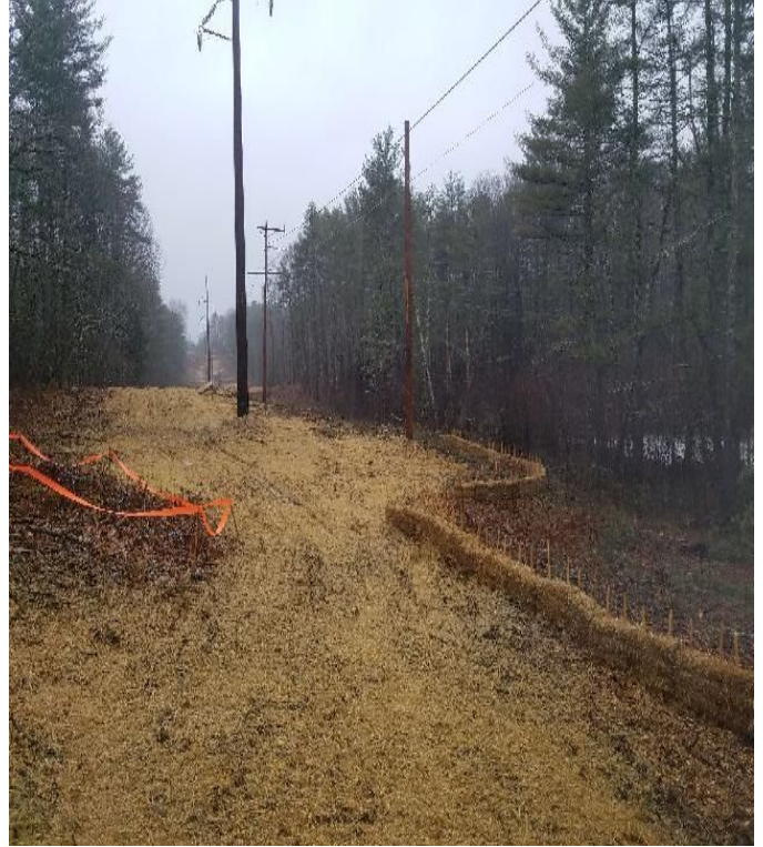
Fig 14: Exposed soils mulched with straw at Str. 62 and 3162-21. Viewing west. (03-13-20).
