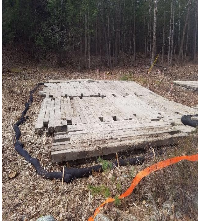
Fig 2: Work pad for Str. 97. Viewing south. (03-12-20).
