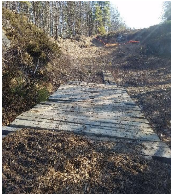
Fig 16: Access road next to wetland DW42, between Strs. 79 and 80. Viewing northeast. (03-16-20).
