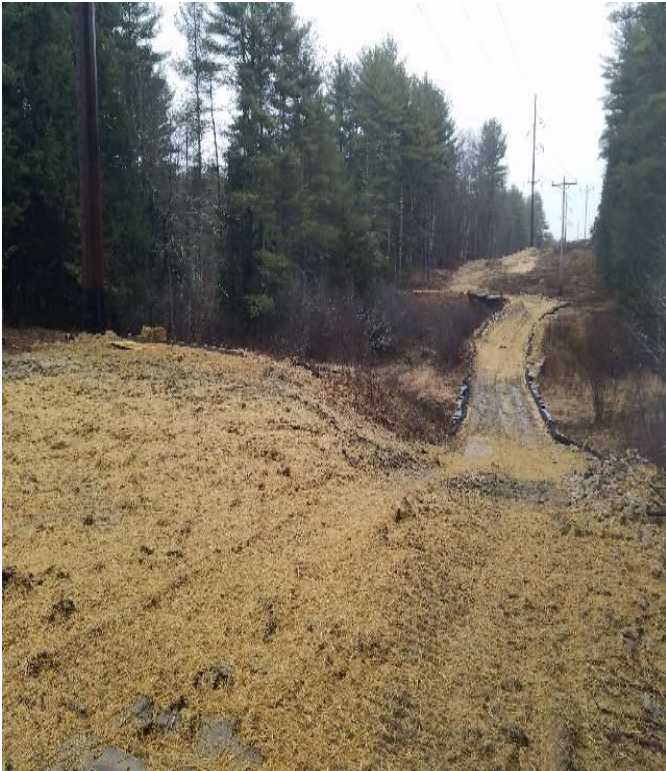
Fig 5: Access road between Strs. 51 and 52, over stream DS46. Viewing east. (03-13-20).
