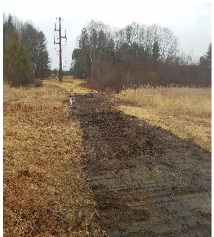
Fig 20: Continue removing timber mats at Frink farm. Viewing west. (03-17-20).
