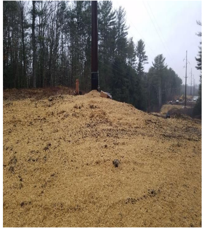
Fig 6: Exposed soils mulched with straw at Str. 52. Viewing southwest. (03-13-20).
