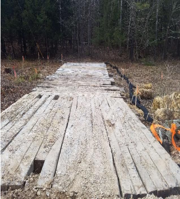
Fig 1: Work pad for Str. 98. Viewing south. (03-12-20).
