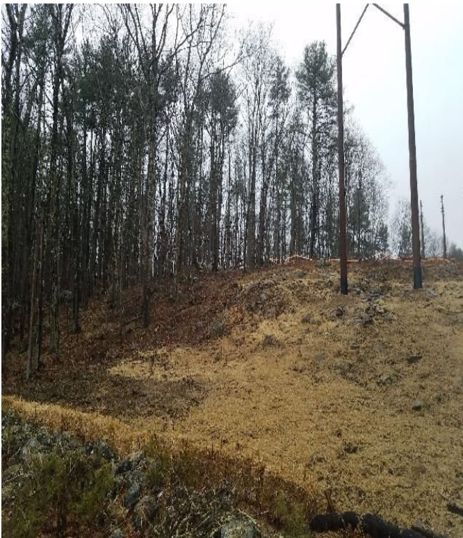
Fig 11: Exposed soils mulched with straw at Str. 57. Viewing northeast. (03-13-20).
