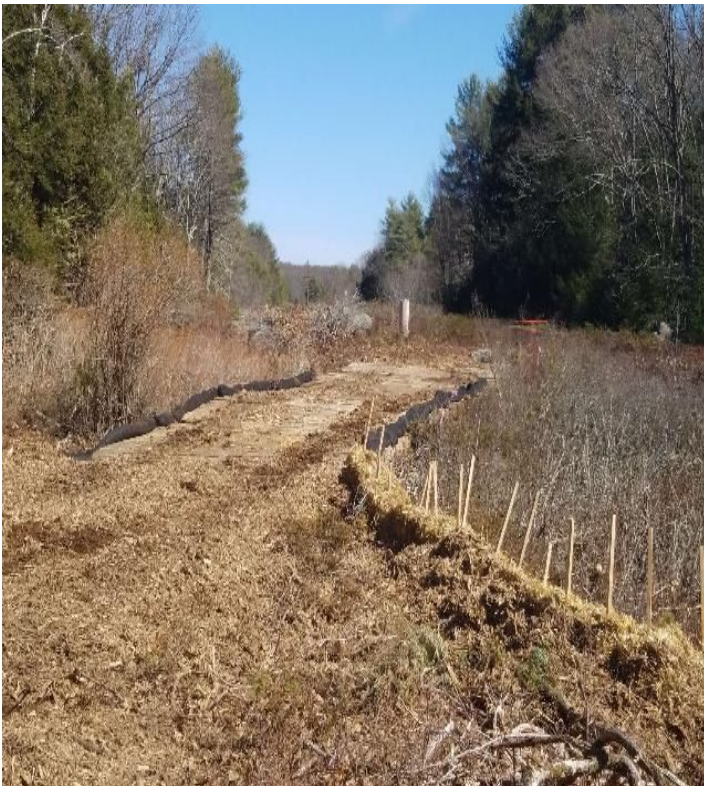
Fig 27: Access road, bridged over wetland DW40. Between Strs 80 and 81. Viewing east. (03-18-20).
